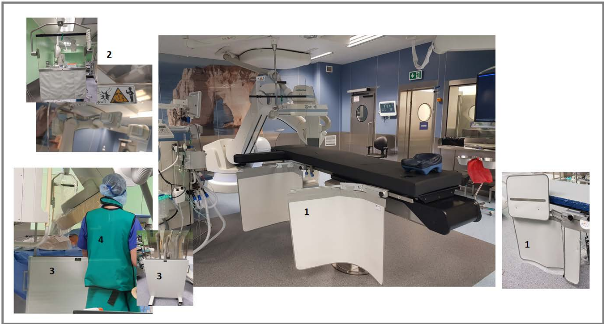
Figure 2. A set of anti-radiation shields in the cath-lab (own figure), 1 — curtain, 2 — ceiling cover, 3 — screen, 4 — personal shields [9]
