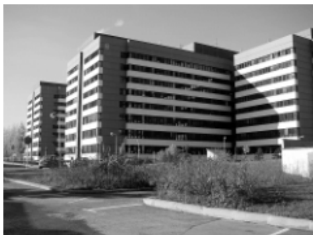
Figure 1. Clinic of Nuclear Medicine, 2 nd Medical School, Charles University Prague in new teaching hospital, Prague Motol.
