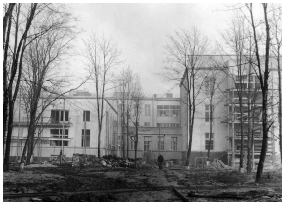
Figure 6. The building of the clinic of the Radium Institute during the completion works, a view from the side of the planned garden (from the collections of the National Digital Archives)
