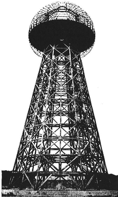
Figure 6. The Wardencliff tower [2]
