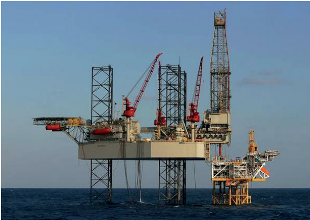
Figure 1. Jack up rig
