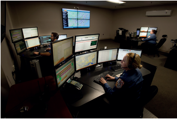
FIGURE 2. JFK control room
